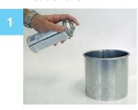
Wipe rolled edge of duct with clean cloth. Then apply a high tack gasket adhesive per the manufacturer's instructions. High tack gasket adhesives can be purchased locally at industrial or automotive suppliers in either aerosol spray or brushable formulations.
