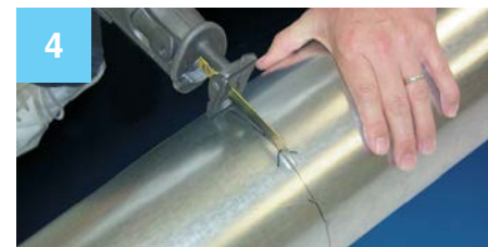
Cut the duct pipe.
