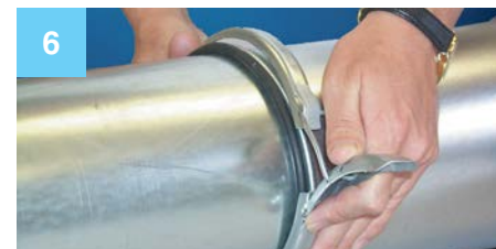
Snap QF clamp over the O-ring and one end of the Adjustable Nipple.
